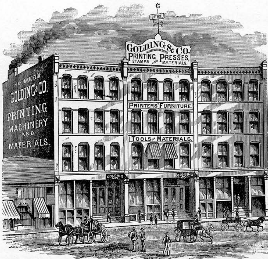
Fig. 8. The Golding factory as it appeared in a wood engraving in the 1884 catalogue of Golding & Co. The building at the left (with smoke pouring from the chimney) is still standing.
